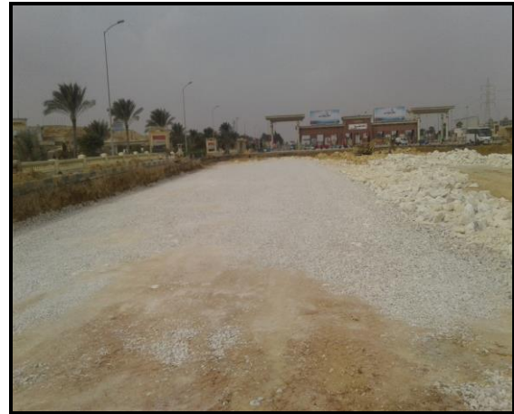
Figure 13. Example of a static steel-wheel roller above filter layer
