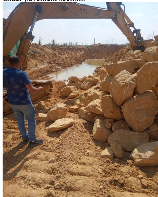
Figure 11. Rock fill for swamp digging bottom
