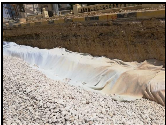
Figure 15. Side Collector filled with geotextile
